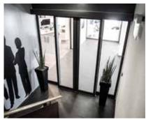
**Sliding fire safety doors** offer both convenient pedestrian access and a resistant barrier in the event of fire. Combined configuration also allows them to function as emergency exits.
