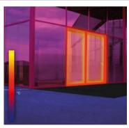
Modern building frontages, let down only by entrances with conventional, non-thermally-insulated profiles = unnecessary loss of energy.
